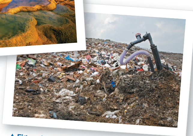
▲ Figure 16.8B Pipes for collecting gas from a landfill
